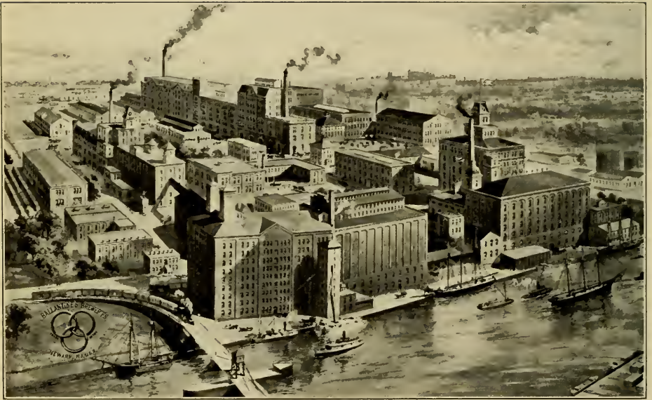
COMBINED VIEW OF BALLANTINE BREWERIES, MALT HOUSES, GRAIN ELEVATOR AND BOTTLER Newark, N. J.
